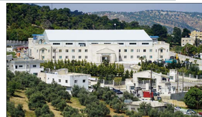
The SESAME building, 35-km north-west of Amman, seen with its new roof in May 2015. (Image credit: CERN-PHOTO-201504-069-15.)
