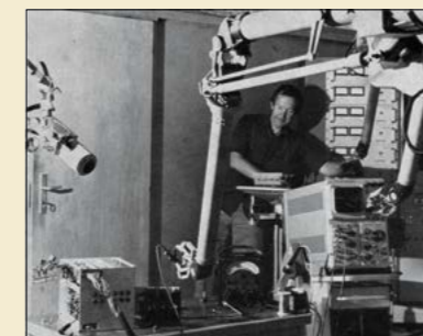
The teleoperator Mascot in action, checking one of its own pulses. Movements of the operator are followed by the slave unit. (Image credit: CERN 99.8.72.)
